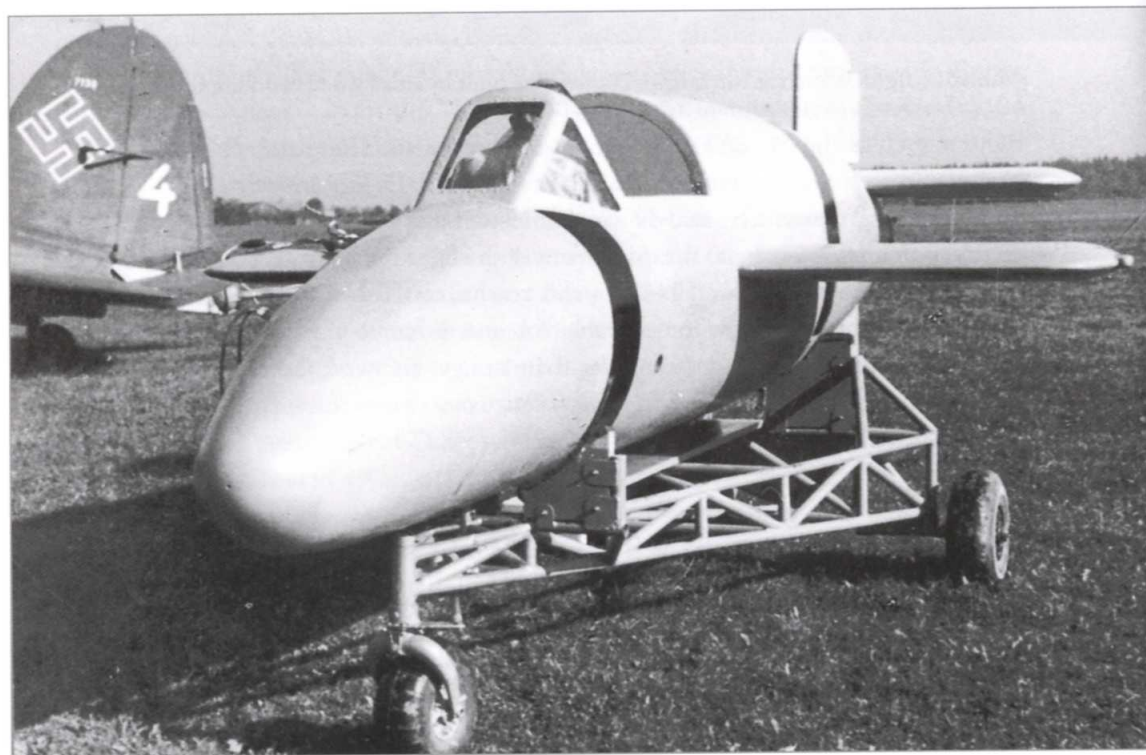
The Bachem Ba 349 Natter was initially flight-tested by the German Research Institute for Gliding as a towed glider.
