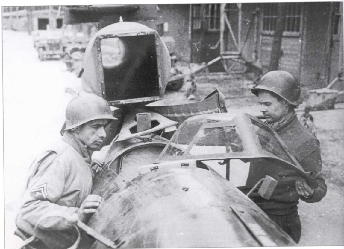
GIs taking a dubious view of the interior of a Fi 103 Reichenberg after removing the cockpit hood.
