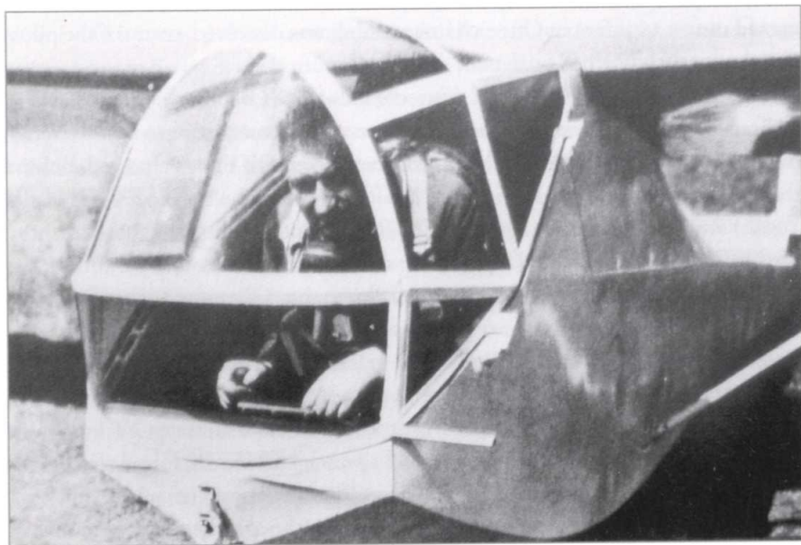
At least one Grunau Baby glider was fitted experimentally with a cockpit in which the pilot could fly the machine in the prone position.
