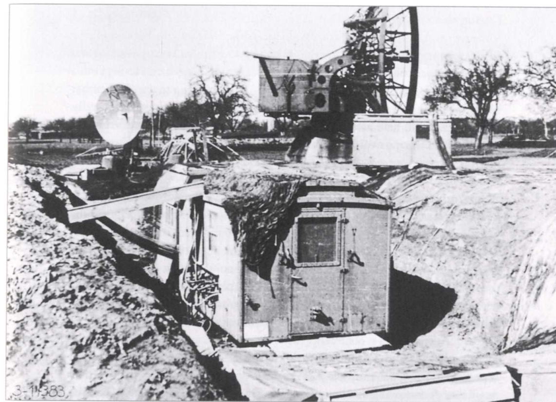
This installation was a test unit for future radars at flak units. On the service vehicle 74/65 can be seen an FuMG 62 Würzburg and an FuMG 65 Würzburg Riese.
