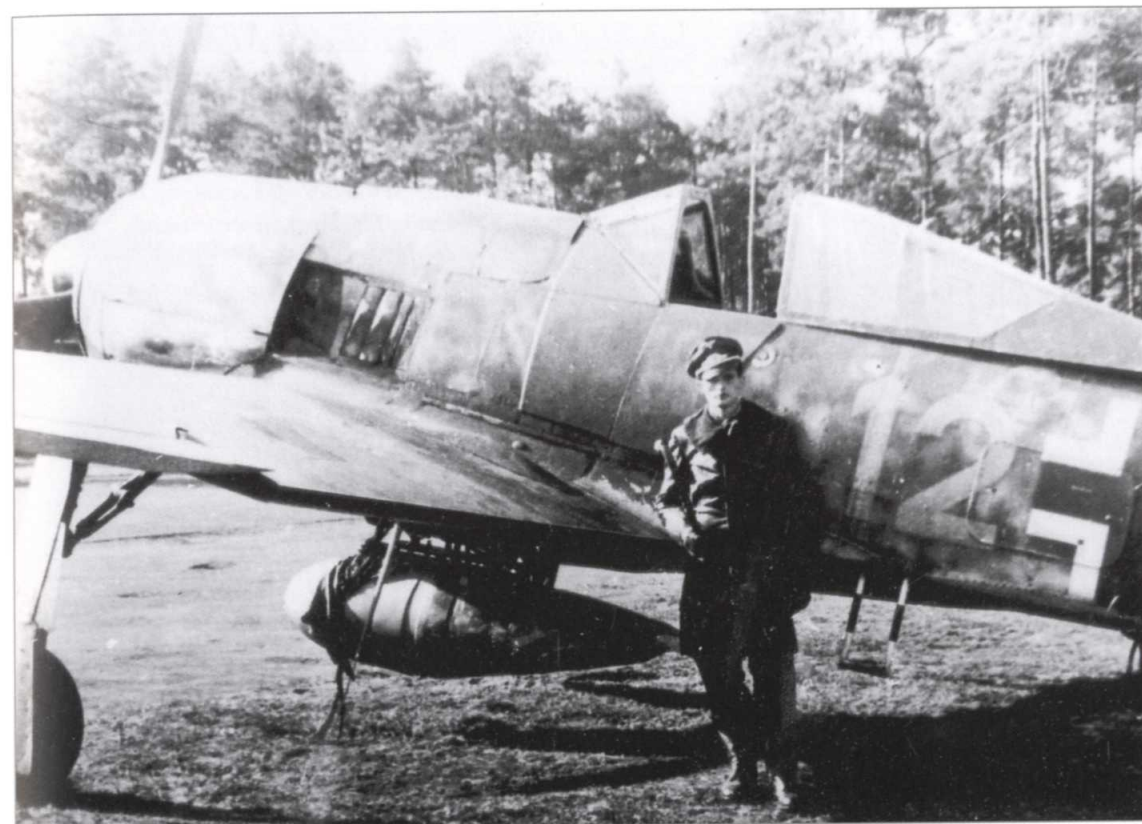
Some Sturmjäger had additional armour on the cockpit sides as can be seen on this Fw 190 A-8.
