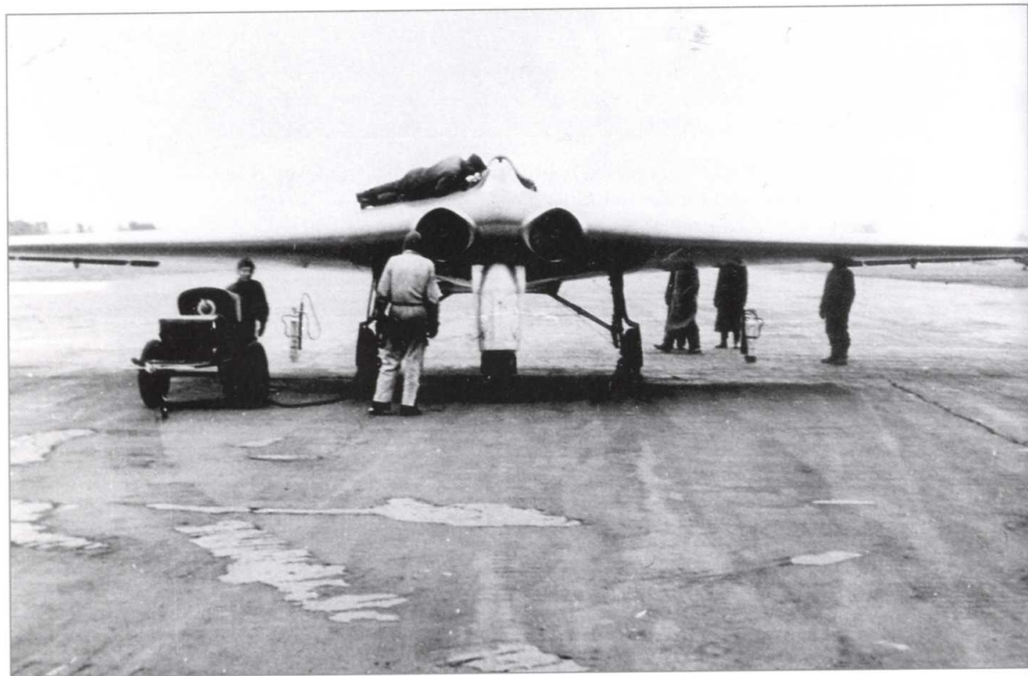
The Horten Ho IX V-2 was driven by two Jumo 004 B jet turbines and tested in February 1945 at Oranienburg near Berlin.
